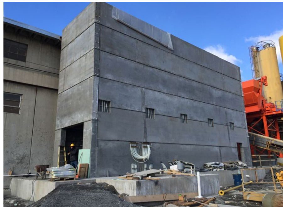
The radiant bunker completed.
