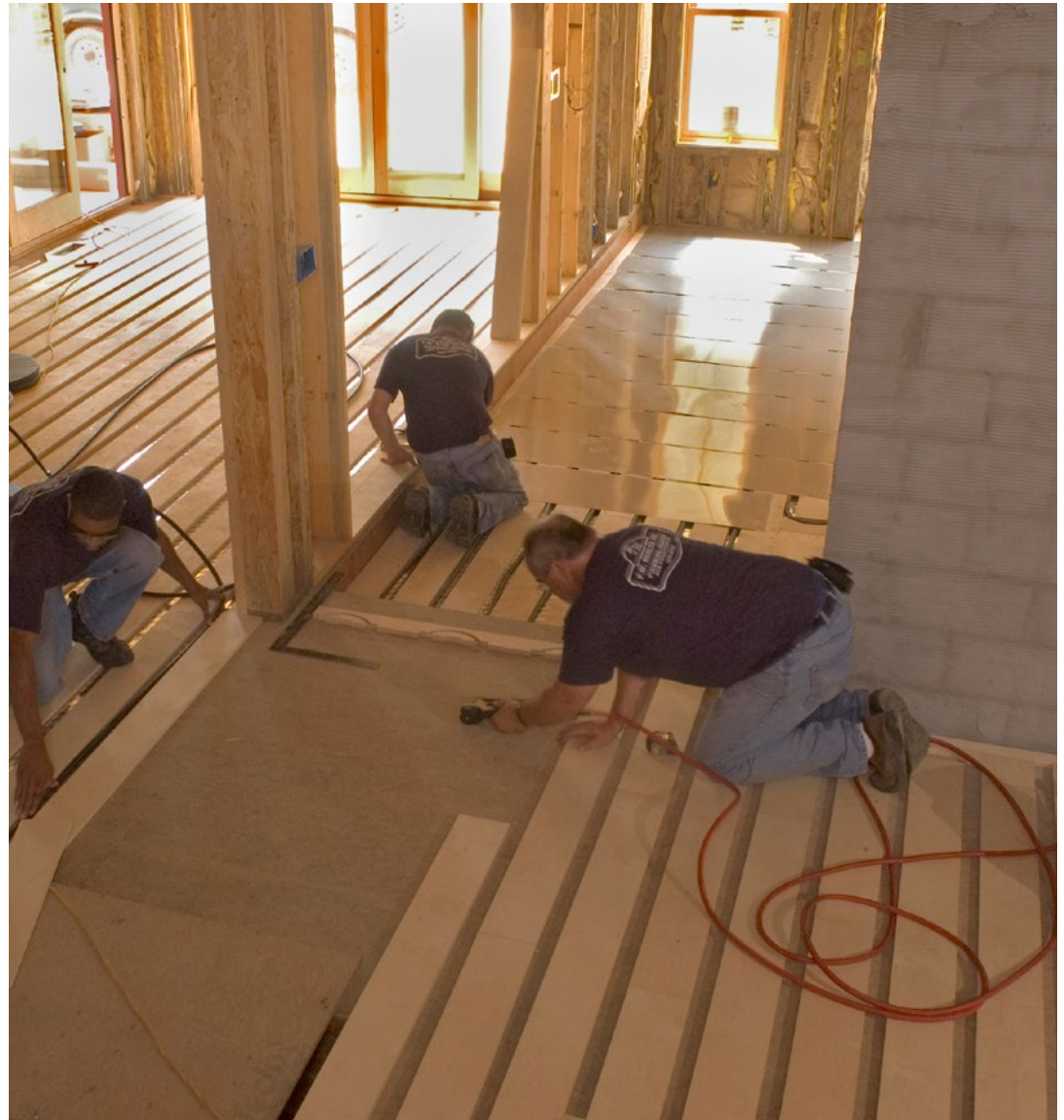
The Behler crew installs Watts SubRay panels, Onix tubing and heat transfer plates.
