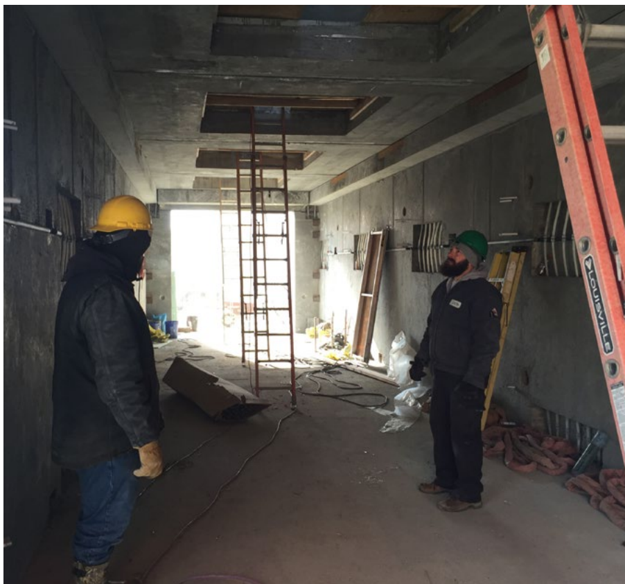
The lower floor of the radiant bunker.
