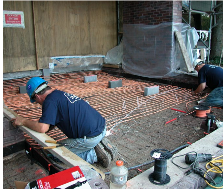
ProMelt cables are installed on the upper landing.
