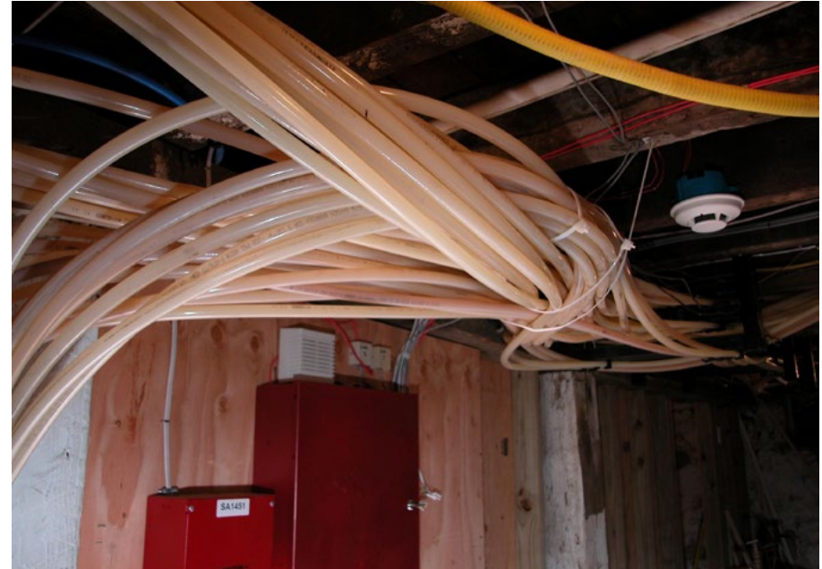
PEX spaghetti held up with plastic strapping that broke.
