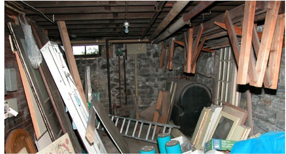
Where's Waldo? A remote antique condensate pump at the far end of the storage room, adjacent to an abandoned oil tank.
