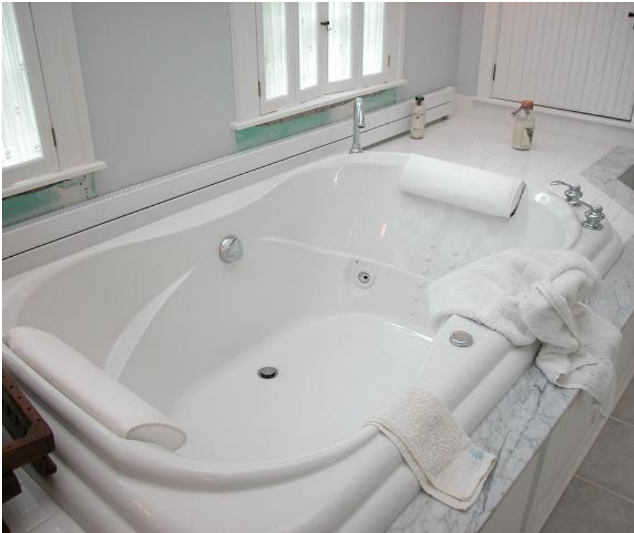
The flat panel radiator to offset chill from adjacent window and supplement heating.
