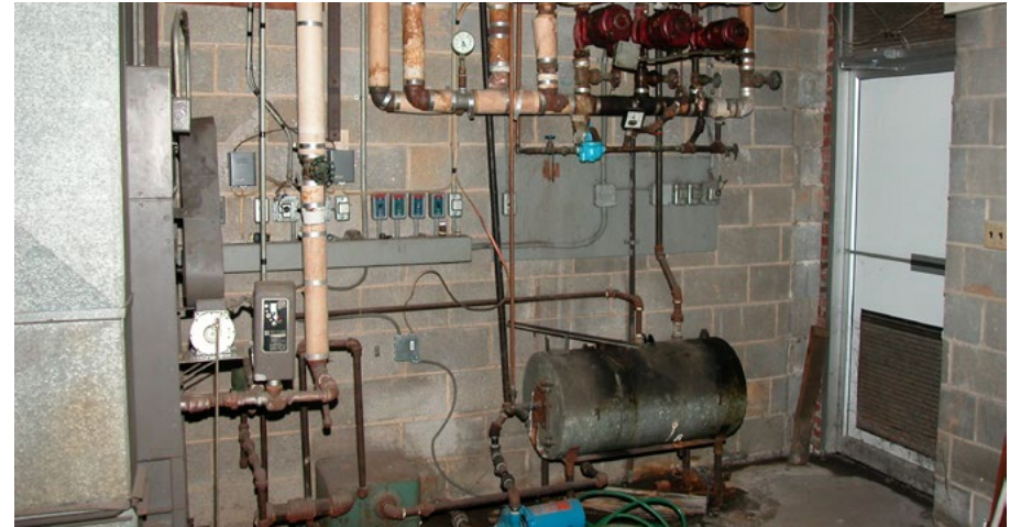
Pictured here is the steam hydro-air on the left; steam condensate receiver/pump and freed-water tank at the bottom right; and hot water distribution piping and circulators at the top right.
