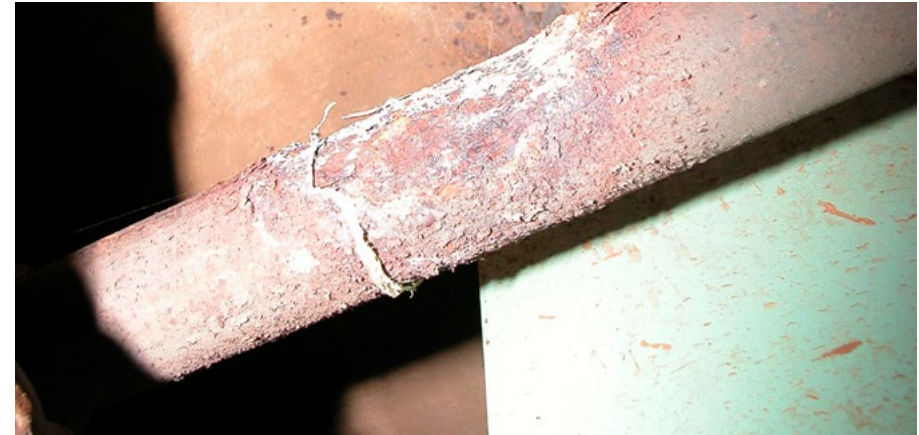
A close up view of acidic condensate damage on a pipe exterior.
