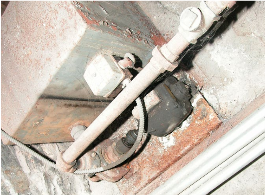
Pipe corrosion from acidic condensate dripping down from open pipe connected to chimney base.
