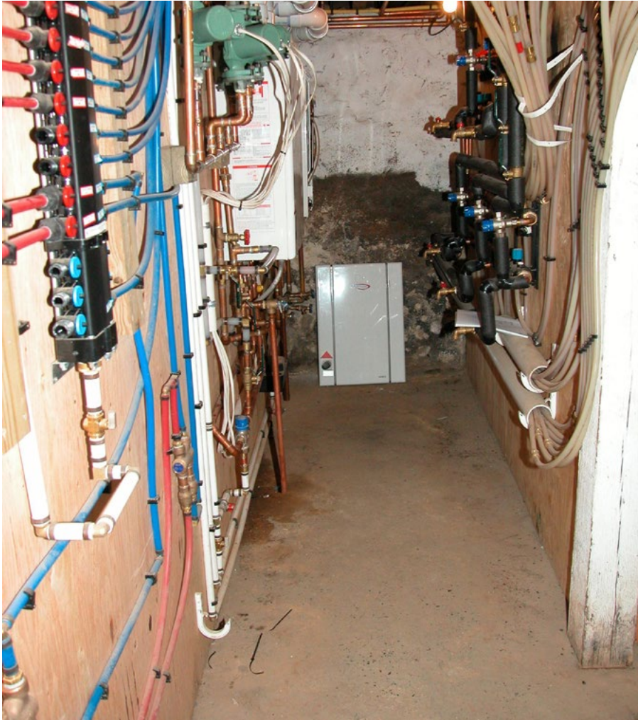
The mechanical nook created very tight quarters.
