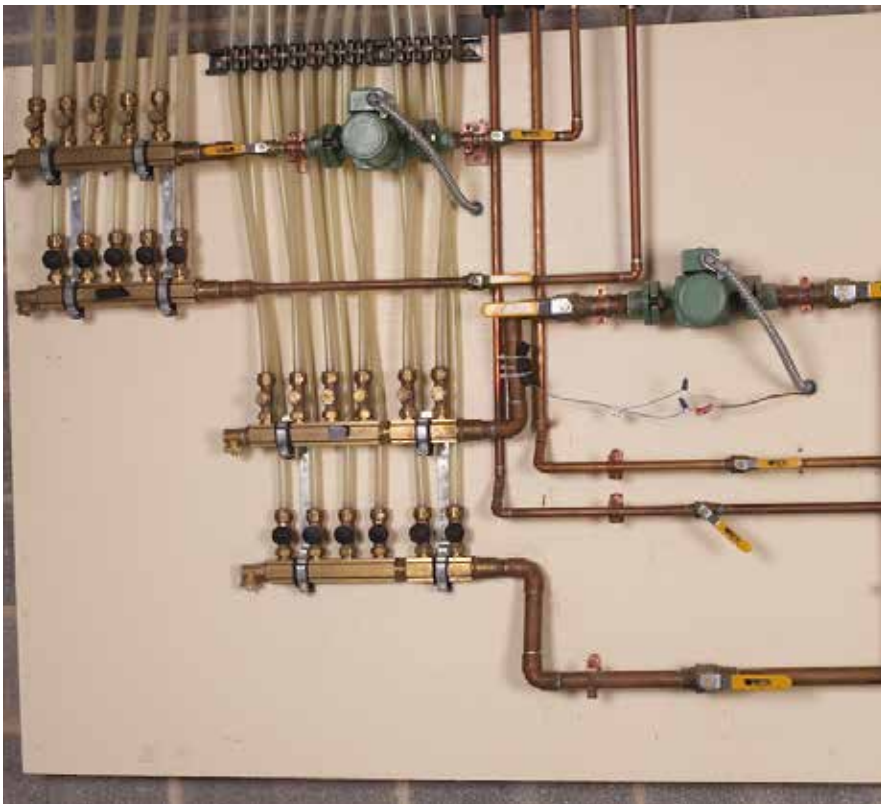
Shop-built injection manifold.
