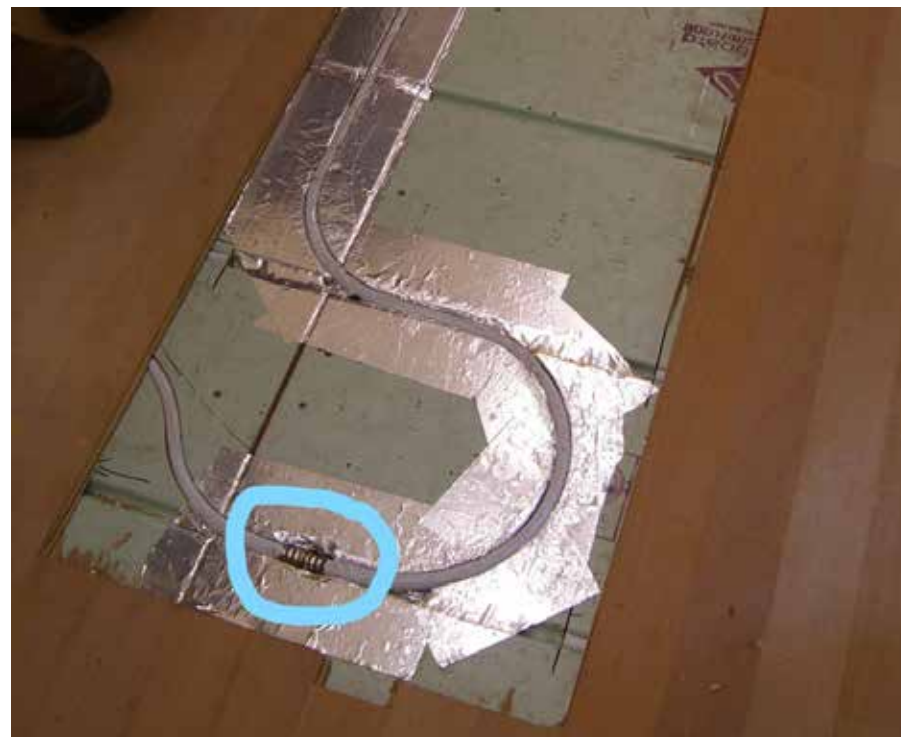
The tubing splice repair fitting is relatively easy to insert.
