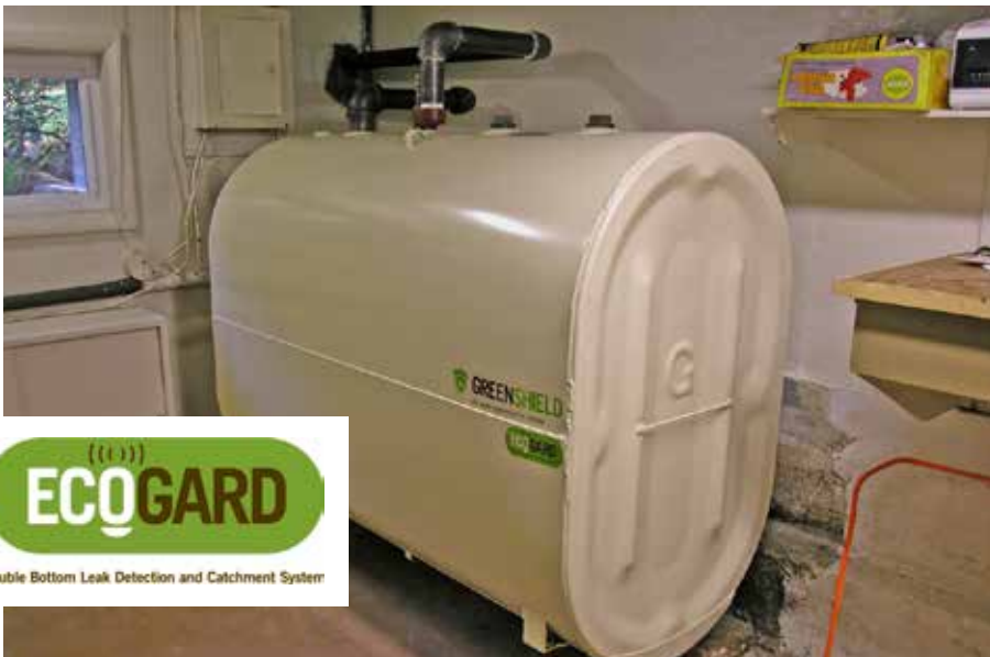
A Granby Greenshield oil tank with double wall safety containment was installed and piping upgraded for code compliance.
