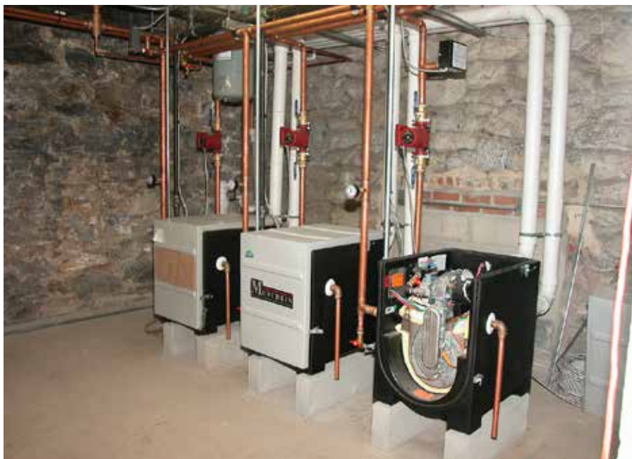
Cascade application of three modulating condensing boilers.
