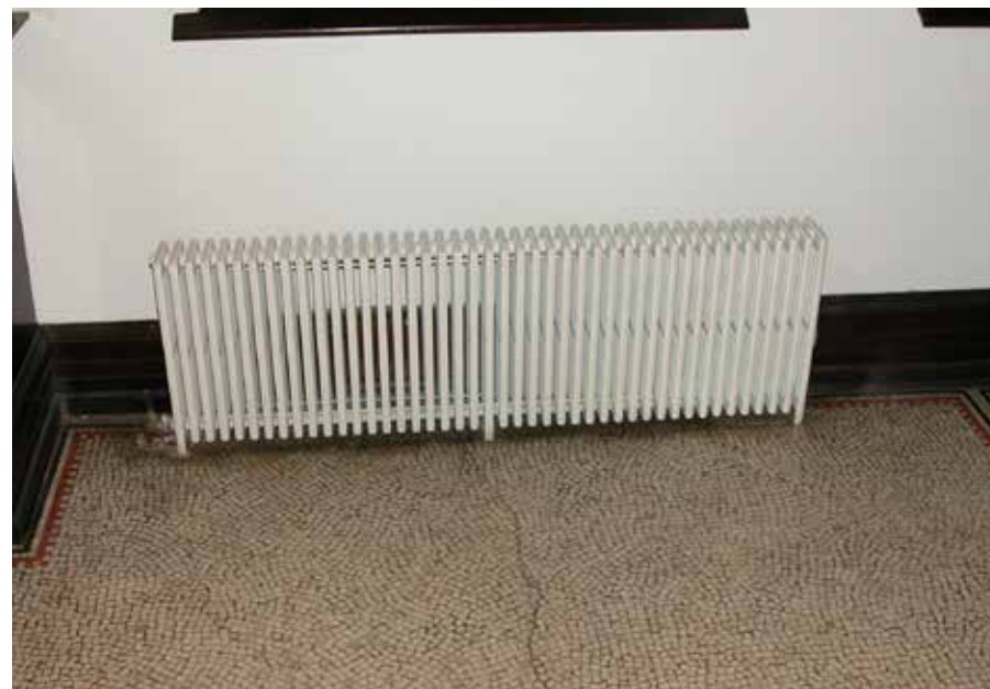
Church radiator converted from steam to gently warmed water.
