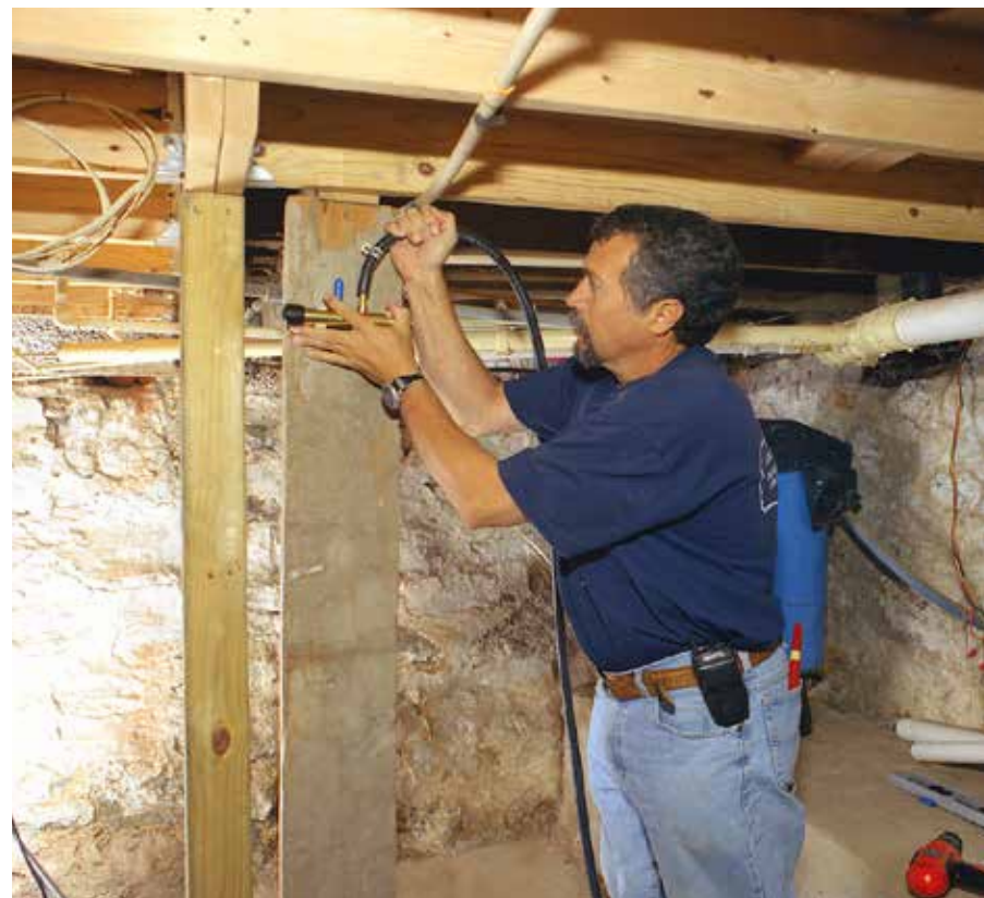
Yates connects Watts Onyx tubing to the zone-to-zone manifold.
