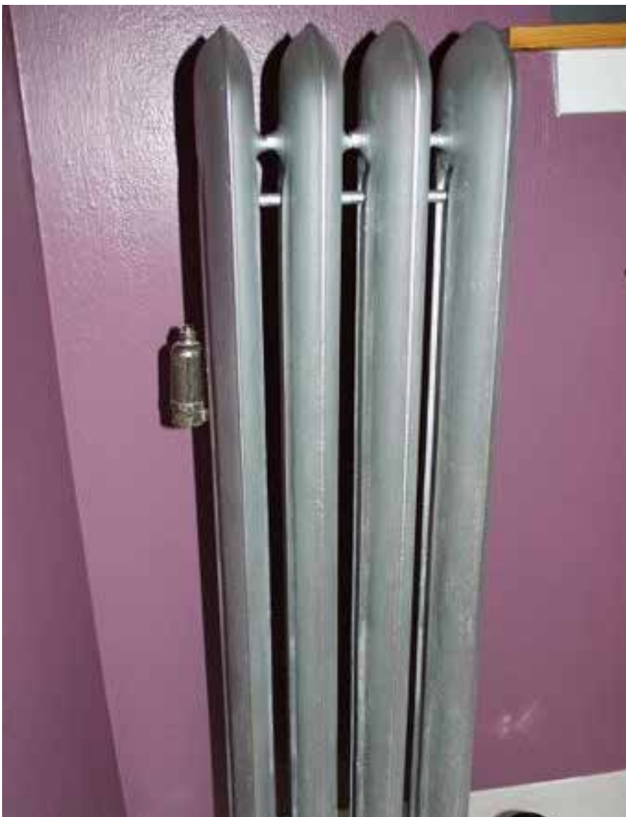
Example of a steam only radiator - no connection between sections near the top.
