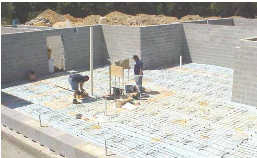
Mike Keefer fastens extruded aluminum heat transfer plated to subfloor.
