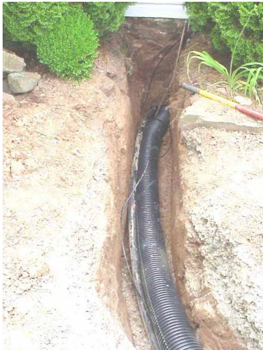
Insulated PEX inside corrugated drainage tube.
