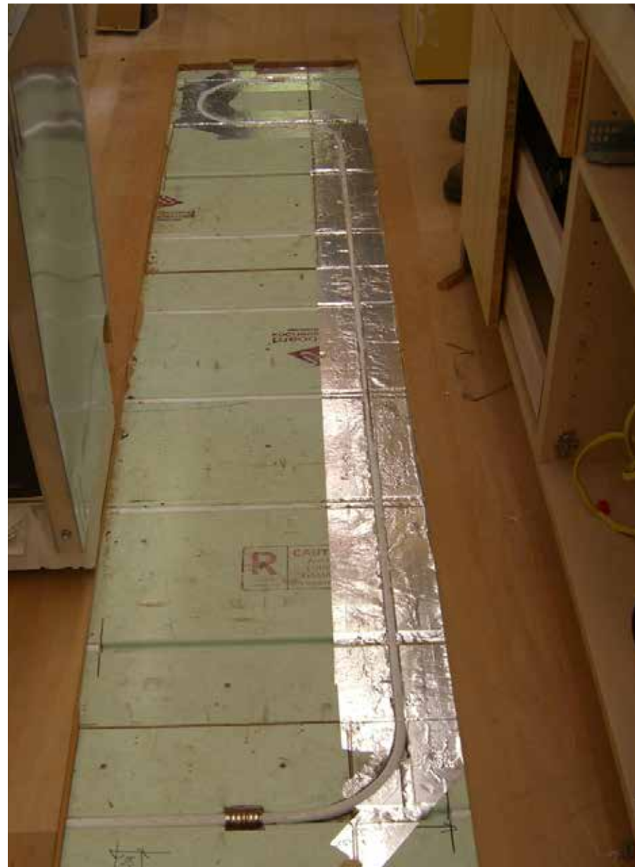
Repair of punctured pex loop.
