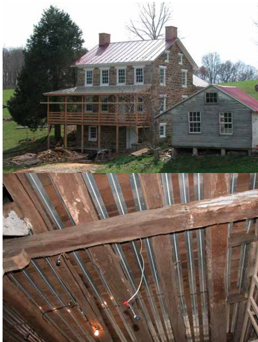
Restored stone farm house where extruded aluminum heat transfer plates were used extensively.
