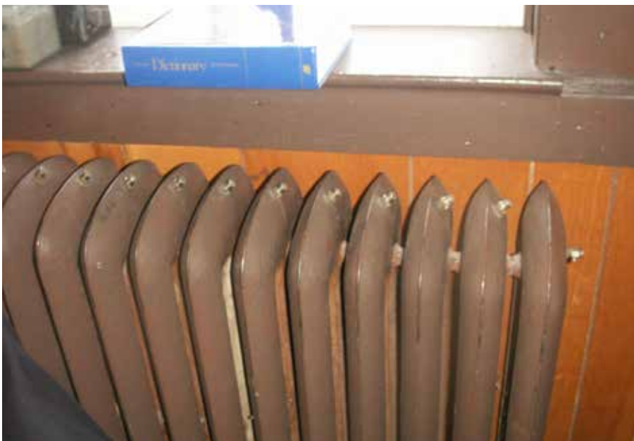
Attempted steam to hot water conversion on a steam-only radiator.
