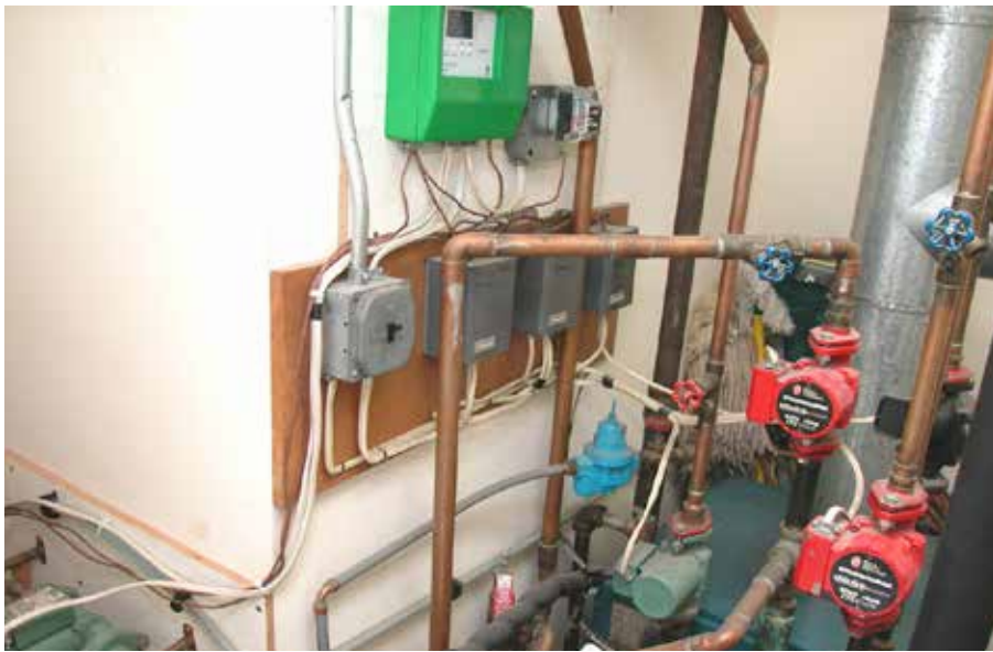
Injection zone added to existing Burnham boiler.
