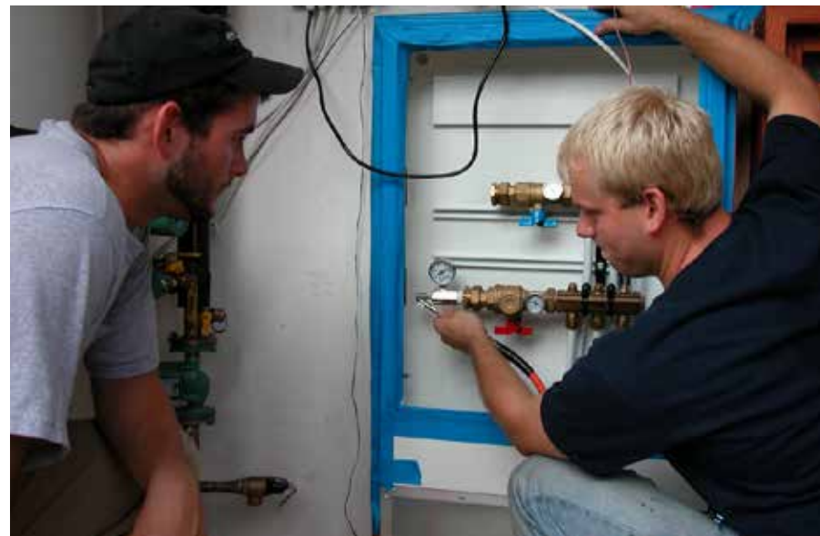
UoM student team members work on assembly of radiant manifold.
