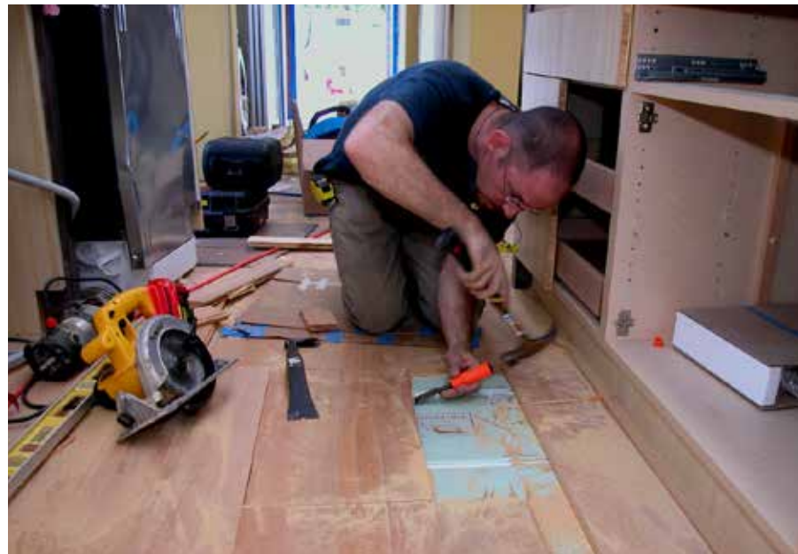
UoM student team member removing Tiger hardwood flooring to expose pex tubing.
