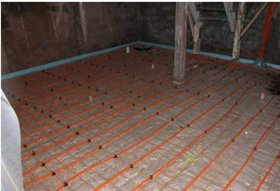
Basement sub-slab PEX loops.
