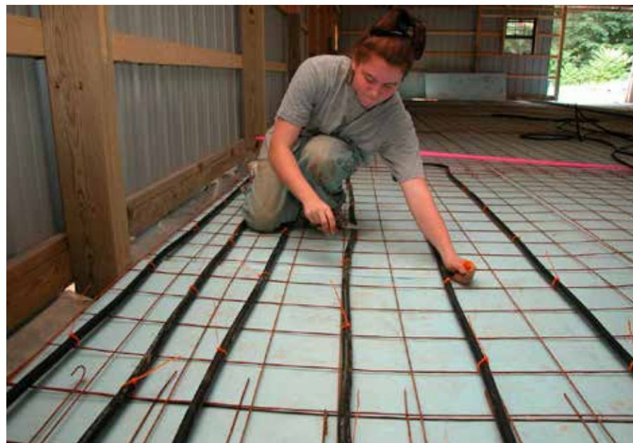
Rehabitat volunteer zip ties Watts Onyx radiant tubing to wire mesh grid.
