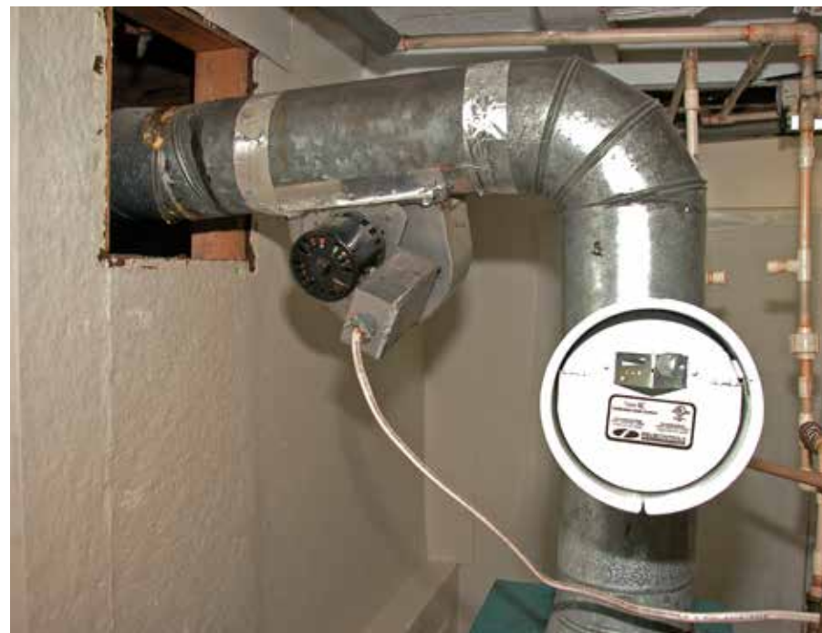
Old boiler's noisy exhaust fan.
