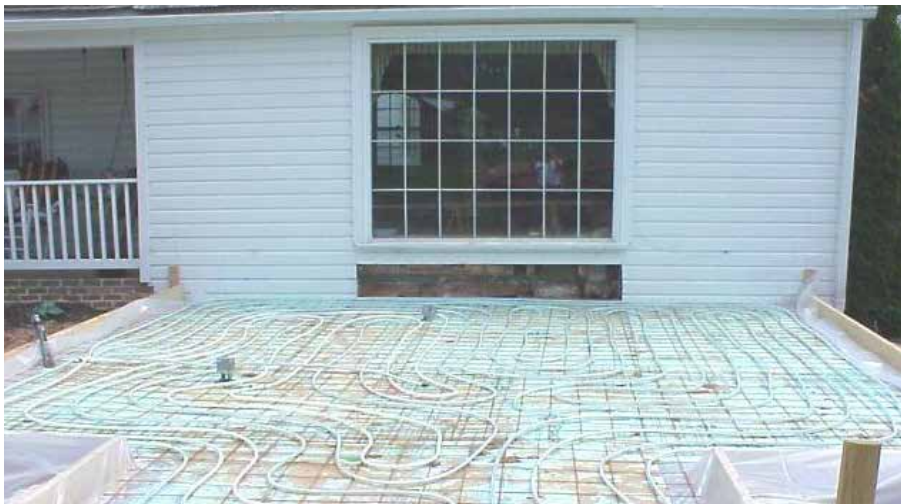
Sub-slab radiant loops of Uponor PEX.
