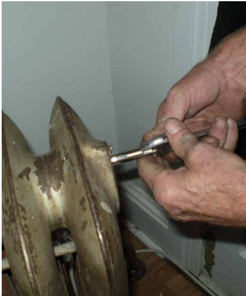
Tapping threads in a radiator to receive a loose key air vent.
