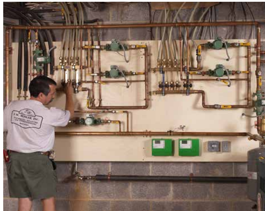
Yates checks manifold performance.
