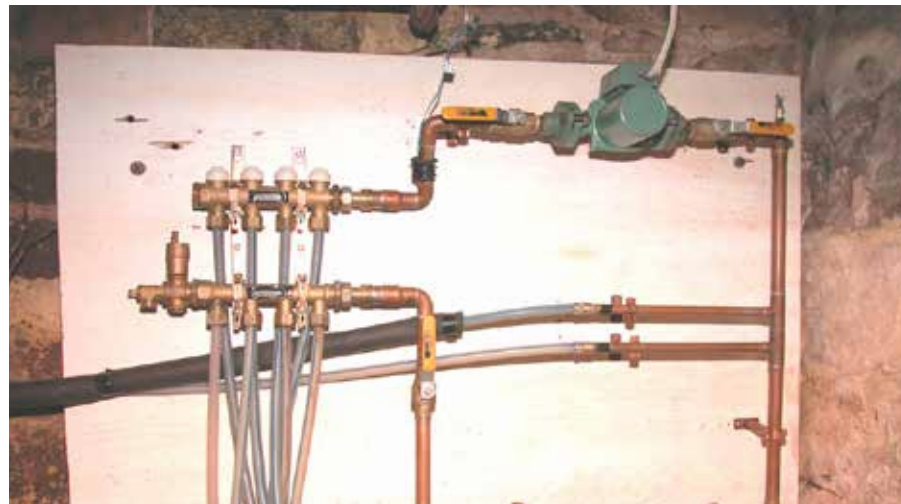
Shop-built injection panel.
