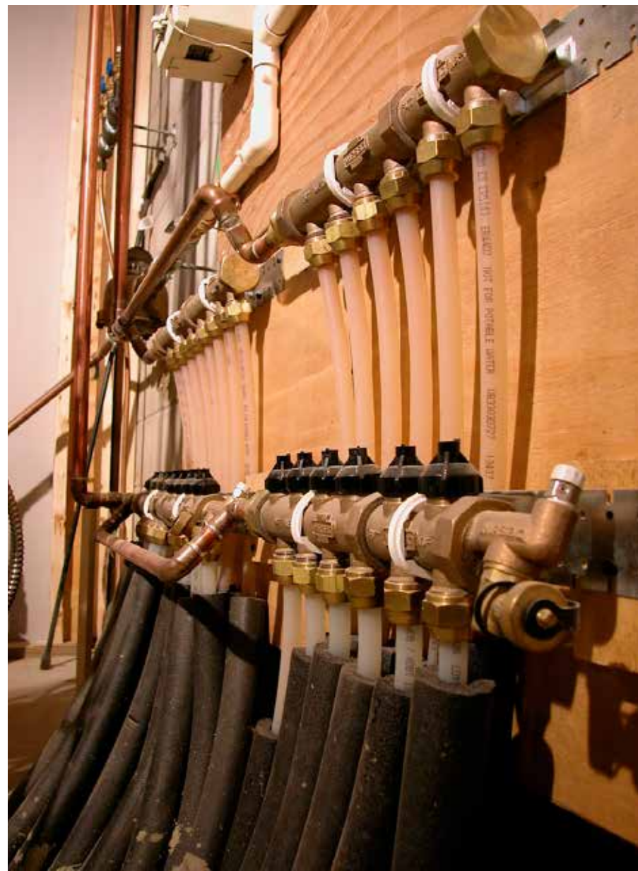
Uponor manifolds piped in reverse-return for balanced flow.
