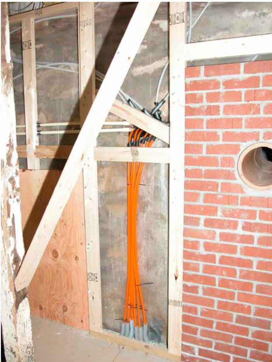
Basement PEX loops after the concrete pour.
