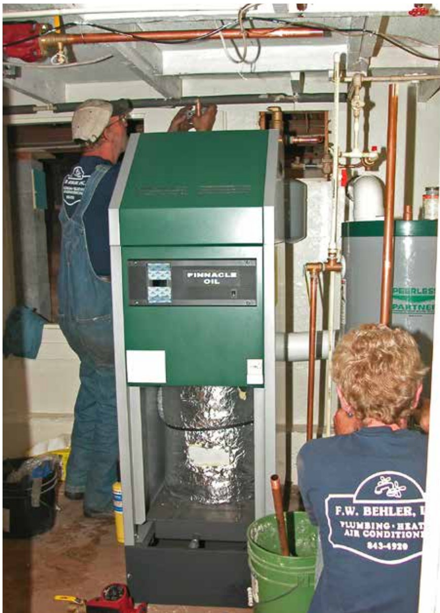
Behler crew installing the Peerless Pinnacle boiler and indirect water heater.
