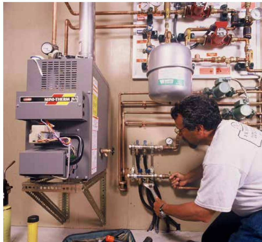
Yates connects a loop of Watts Onix barrier tubing.
