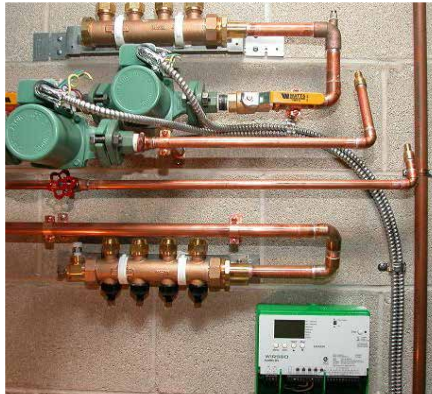
Remote manifolds: one direct and one injection.
