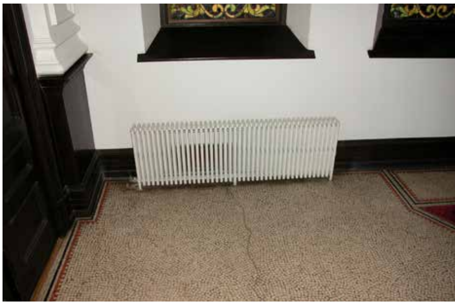
Steam radiator in Sanctuary converted to use gently warmed water.
