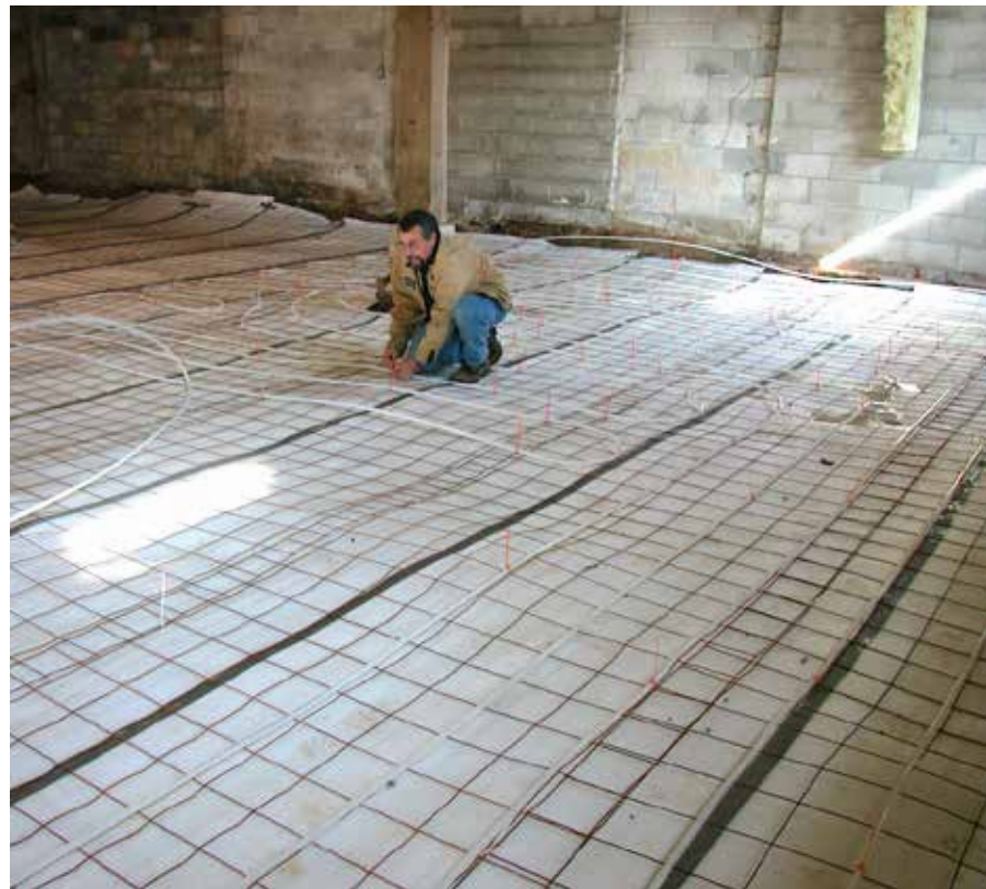
Yates fastens Uponor barrier PEX tubing to wire mesh grid.
