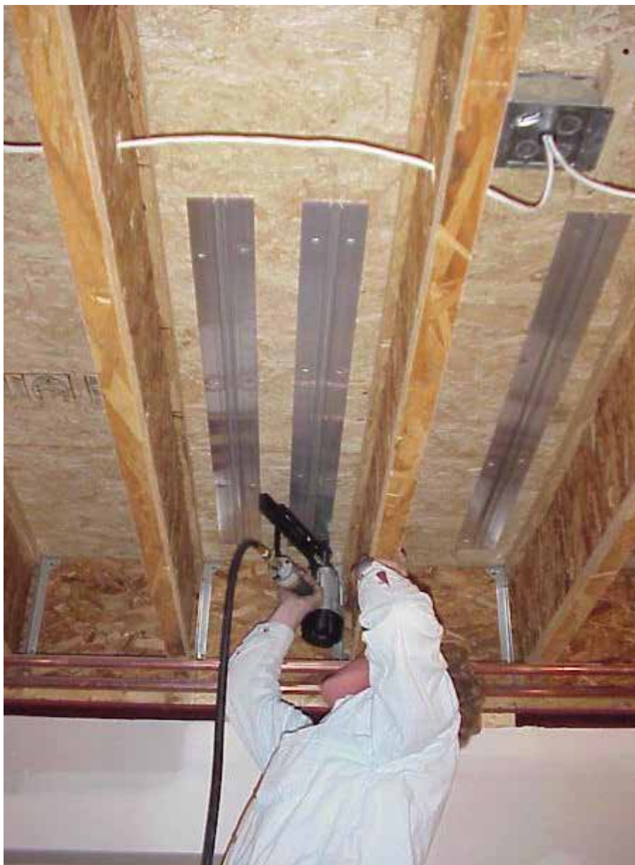
Mike Keefer fastens extruded aluminum heat transfer plated to subfloor.
