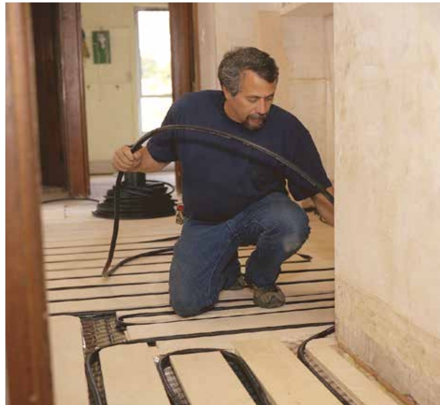
Yates placing Watts Onyx barrier tubing in Subray tracks.
