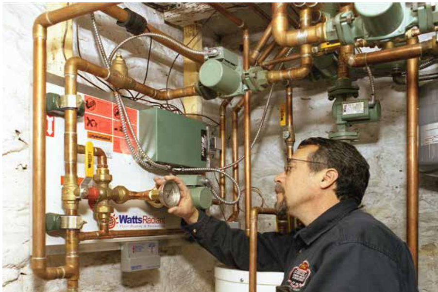
Yates checks water temperature on the Watts-built controller panel.
