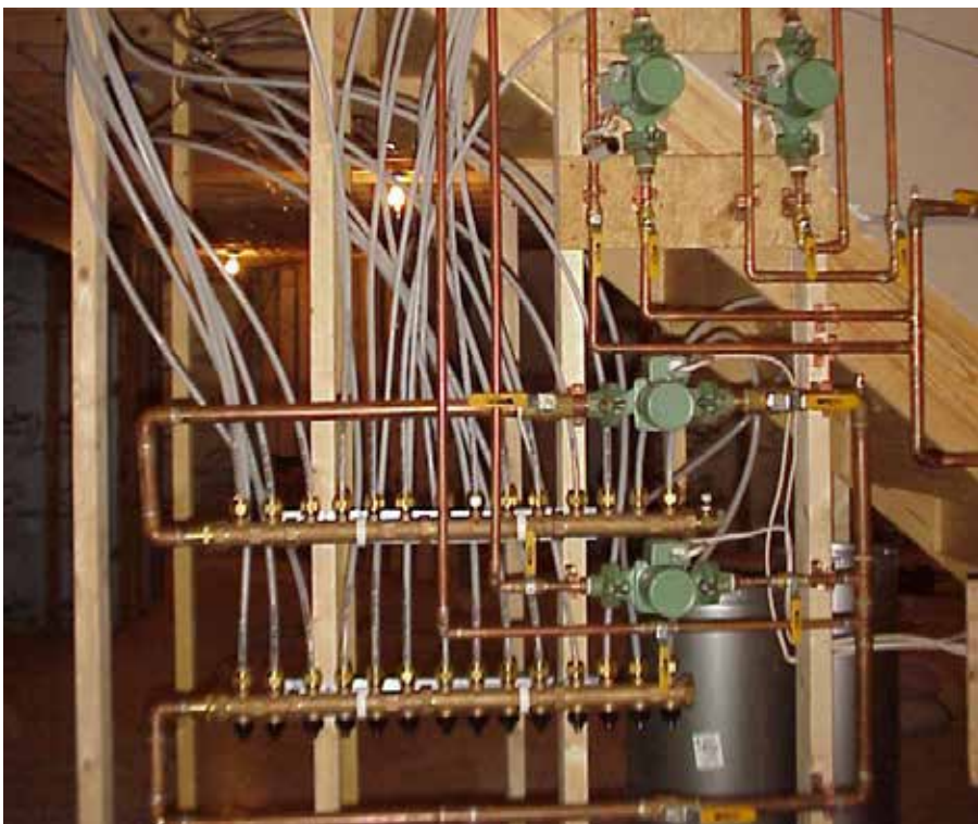
After the Behler crew installed manifolds, Hanson connected the Uponor PEX reverse-return loops.
