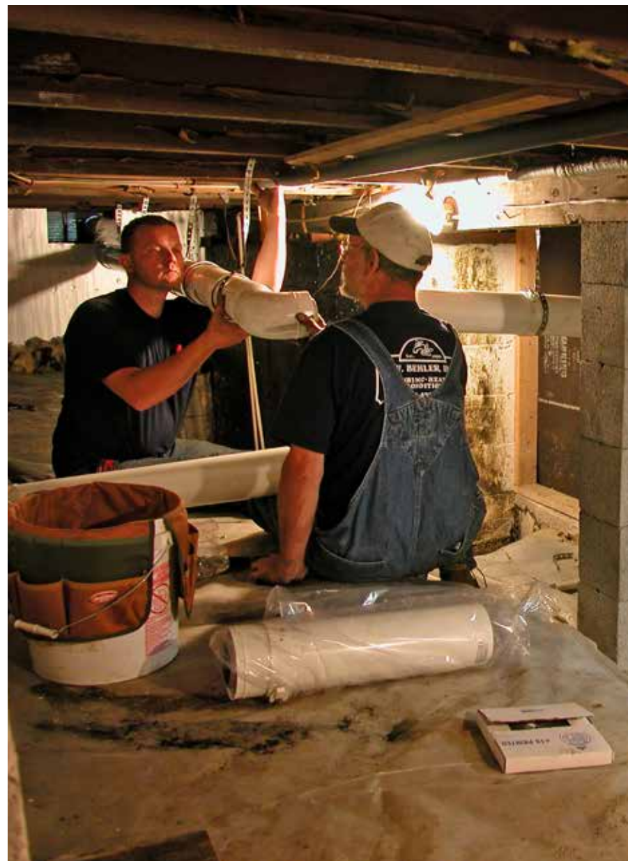
Installing the Peerless pipe-in-pipe I take/exhaust flue piping.
