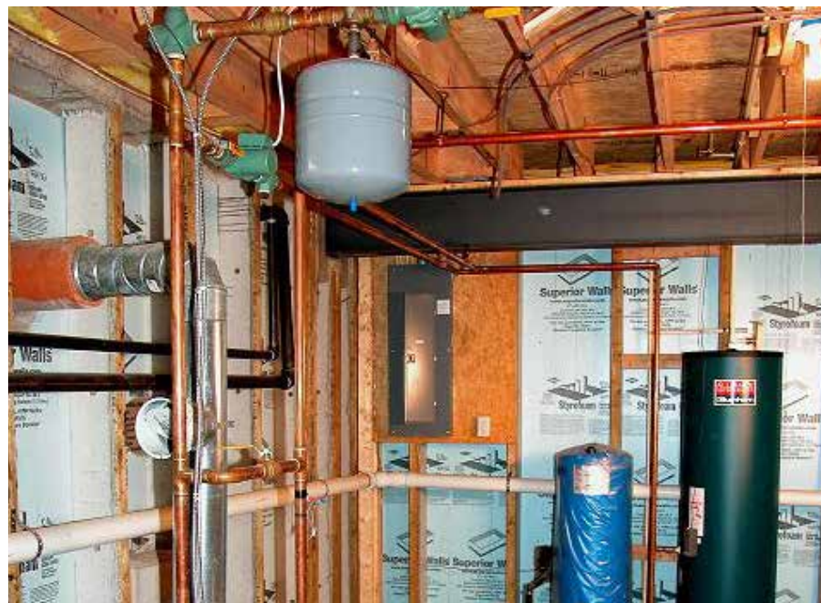
Hydronic piping included a boiler bypass line.
