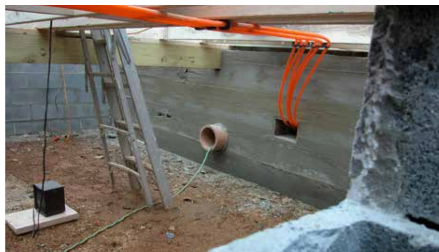
PEX tubing on its way to the basement zone.
