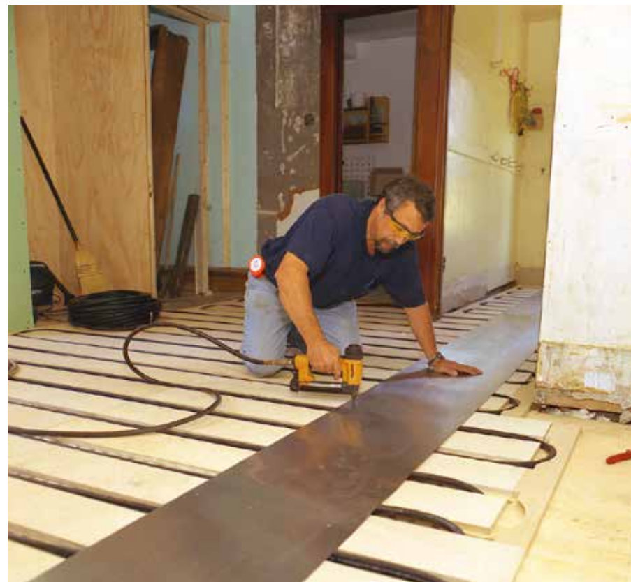
Yates tacks down aluminum heat transfer sheet over Watts Subray panels.
