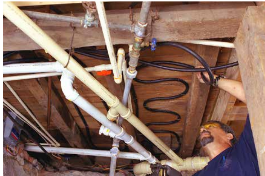
Yates installing Watts Onyx barrier tubing.
