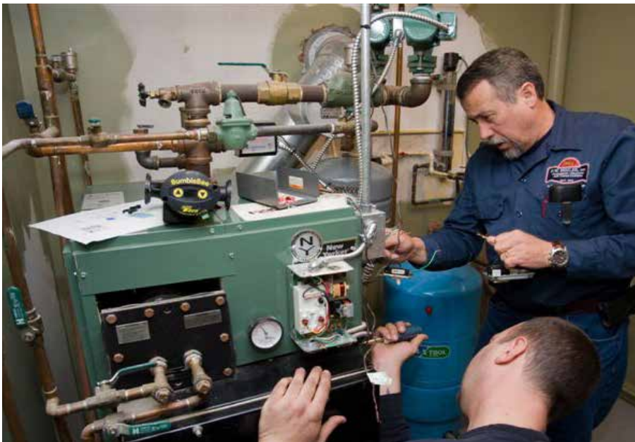
Dave Yates and Larry Lawrence dismantling the old boiler.
