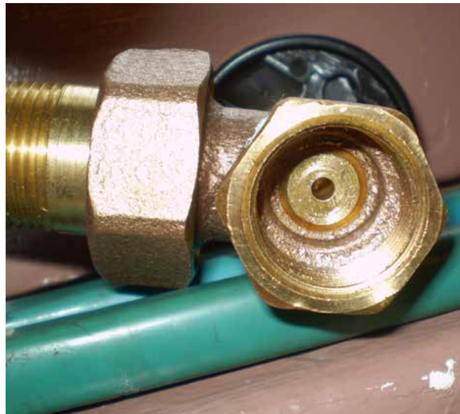
Hot water radiator valve with weep hole.
