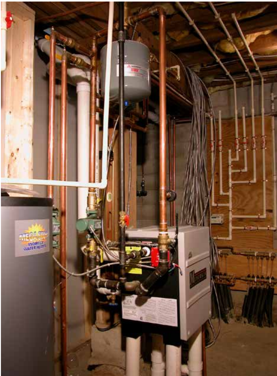
Popane-fired modcon boiler with indirect water heater.
