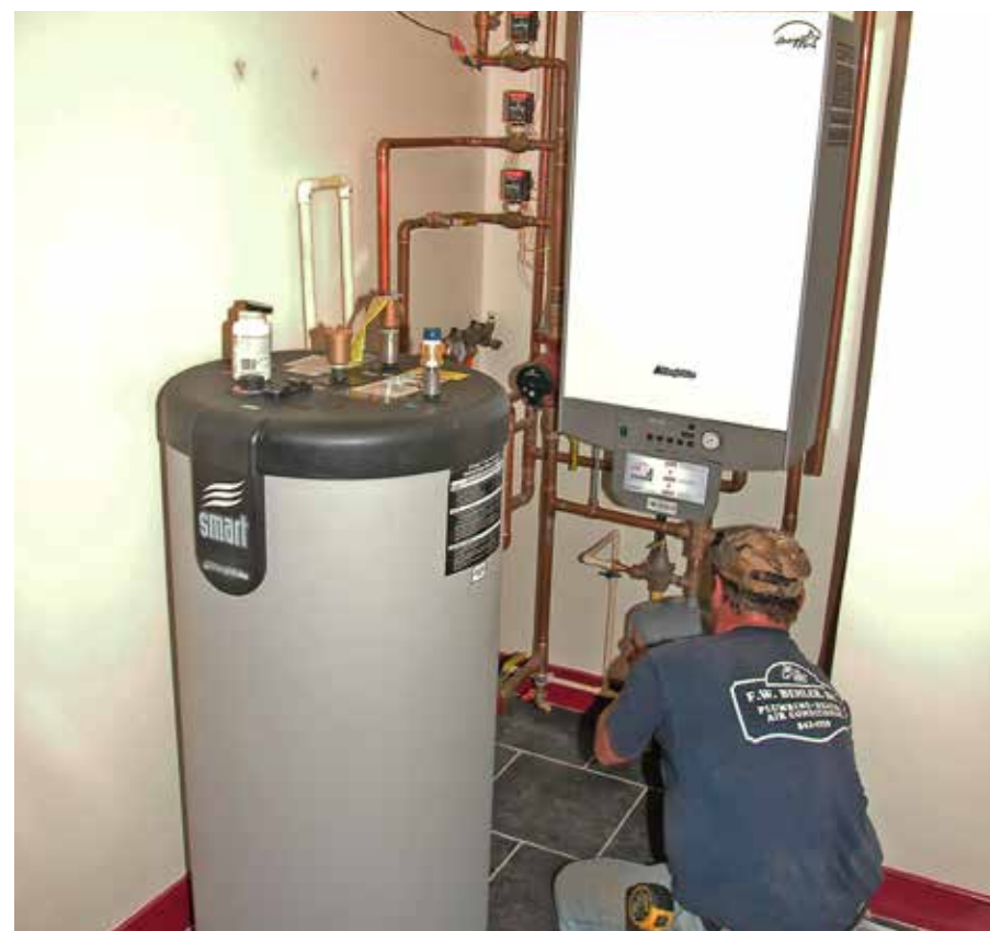
Triangle Tube modcon boiler with Smart 40 indirect water heater.
