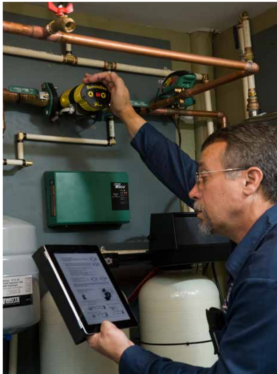
Yates programming the Taco ECM circulator.
