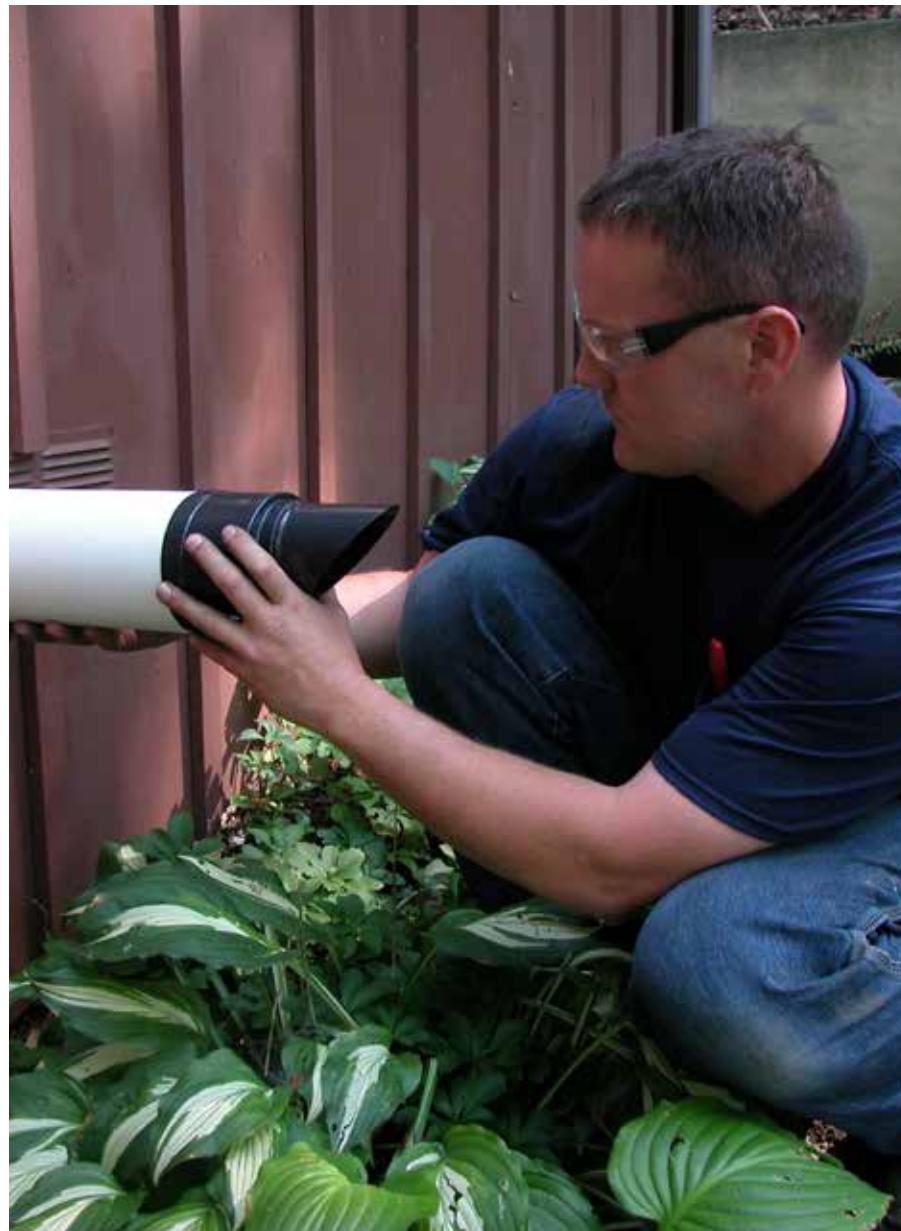
Installation of the Peerless dual intake/exhaust flue pipe.
