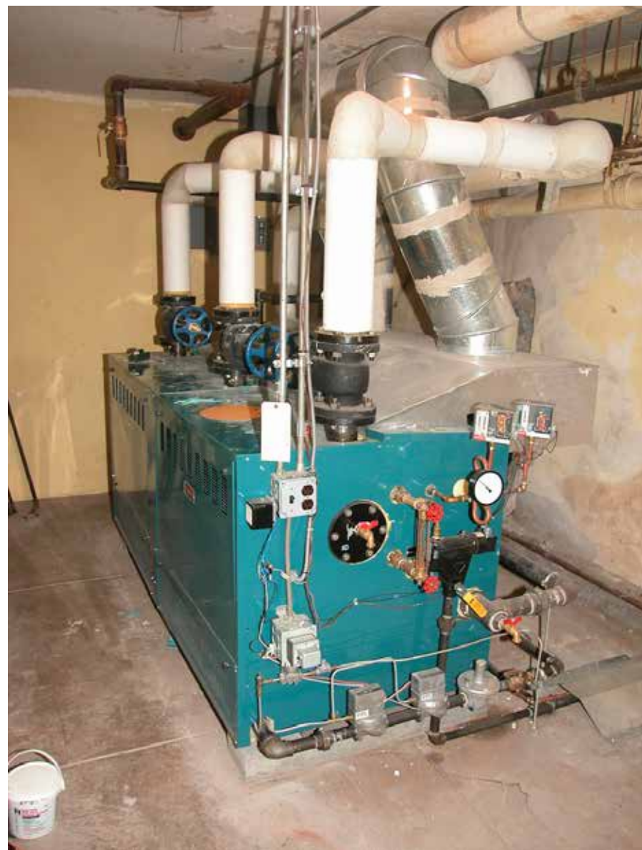
New properly sized Burnham steam boiler.
