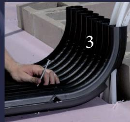
Notice in the picture to the left that by cutting the back-underside of the Premier, you have the option to run lines from other directions.
