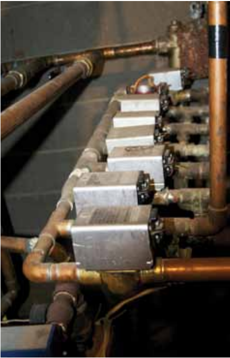
The fin-tube radiation enclosure in an apartment had a manual damper that was almost closed on top. Once the damper was opened wide, the heat convection was felt immediately.
